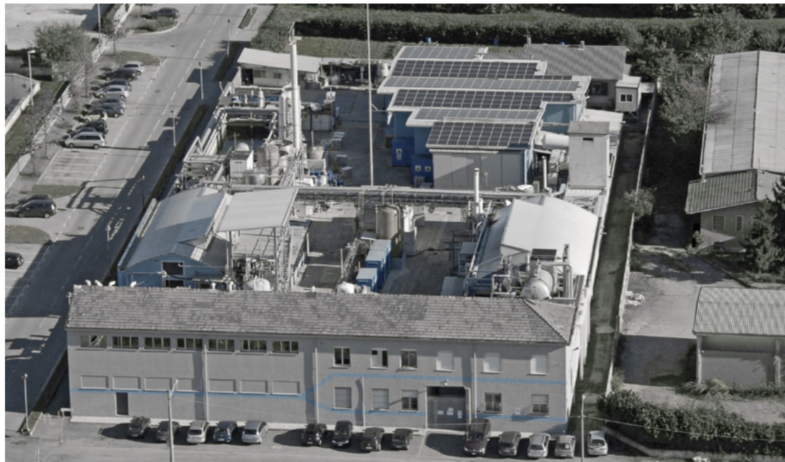
ICROM FACILITIES YEAR 2004
